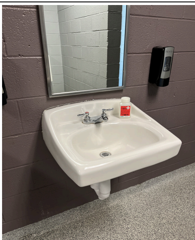
3/12/2024 - 5801-48 - Midway R-1 - Men's Restroom Across From 406 - Closest To Door
