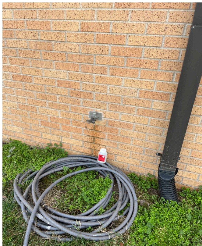
3/12/2024 - 5801-83 - Midway R-1 - Exterior Outside Room 319
