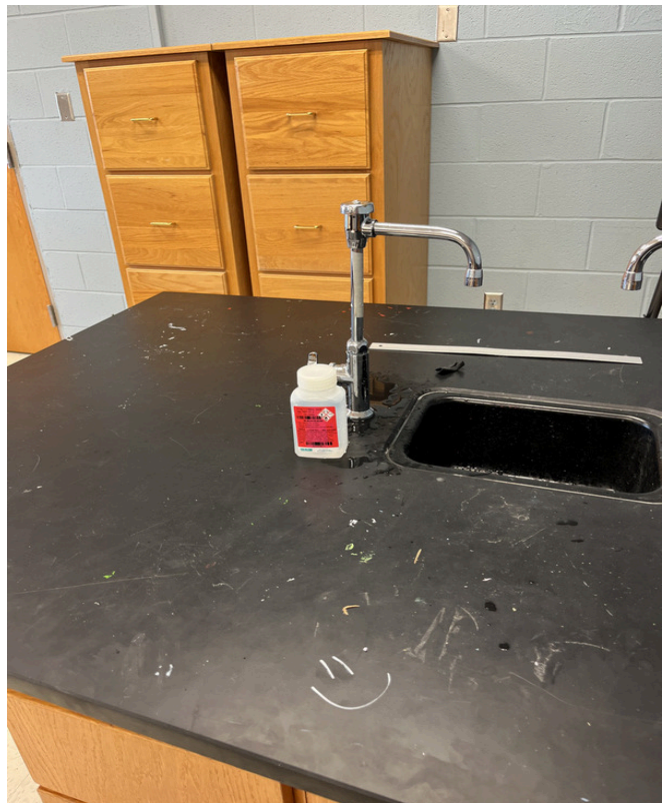
3/12/2024 - 5801-37 - Midway R-1 - Room 202 - North Side - Third Row - Left Faucet
