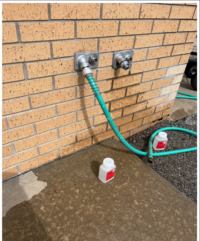
3/12/2024 - 5801-90 - Midway R-1 - North Exterior Outside Room 210 - Left
