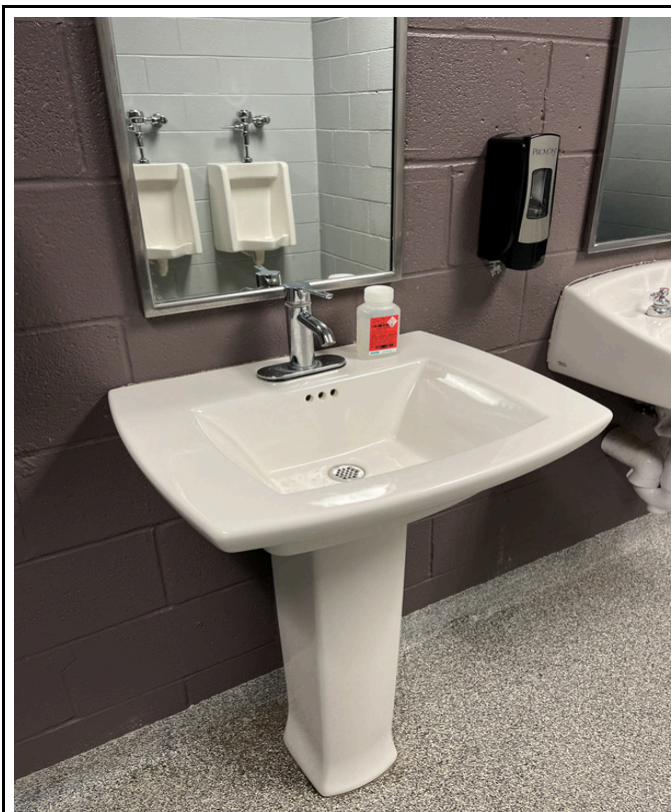
3/12/2024 - 5801-47 - Midway R-1 - Men's Restroom Across From 406 - Furthest From Door
