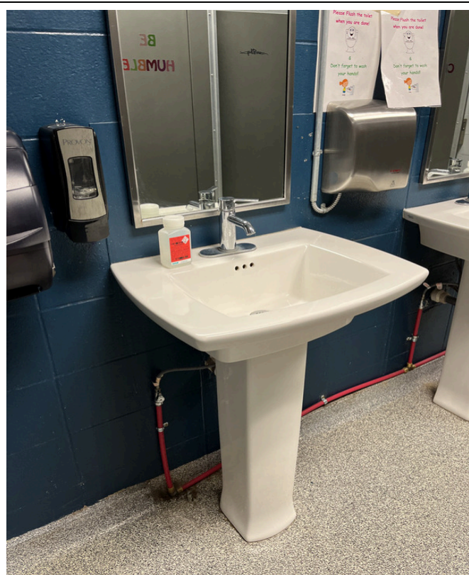
3/12/2024 - 5801-7 - Midway R-1 - Women's Restroom Outside 307 - Closest to Door
