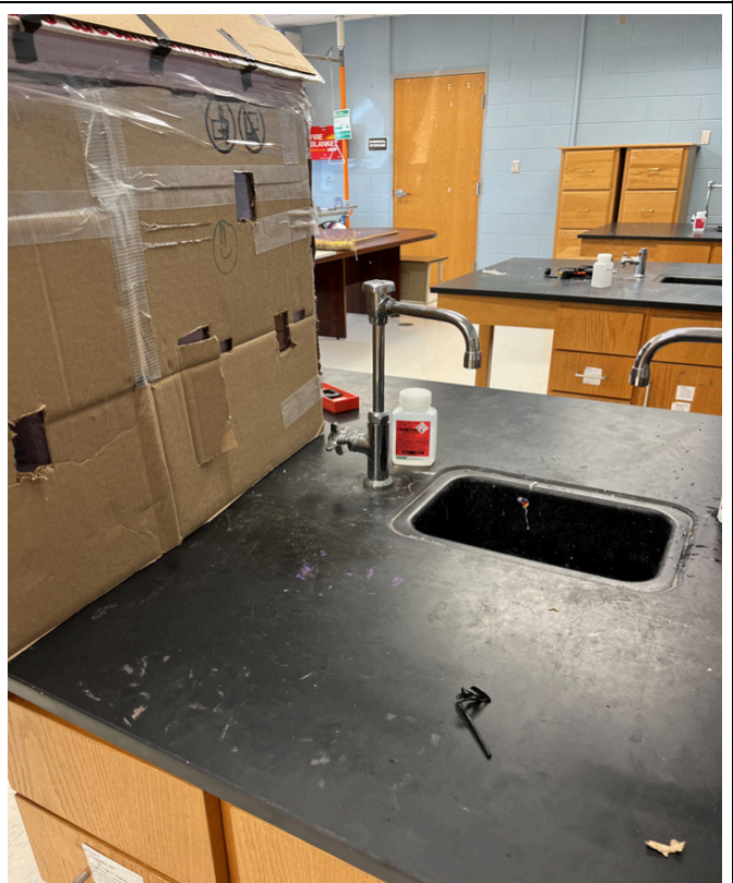
3/12/2024 - 5801-33 - Midway R-1 - Room 202 - North Side - First Row - Left Faucet
