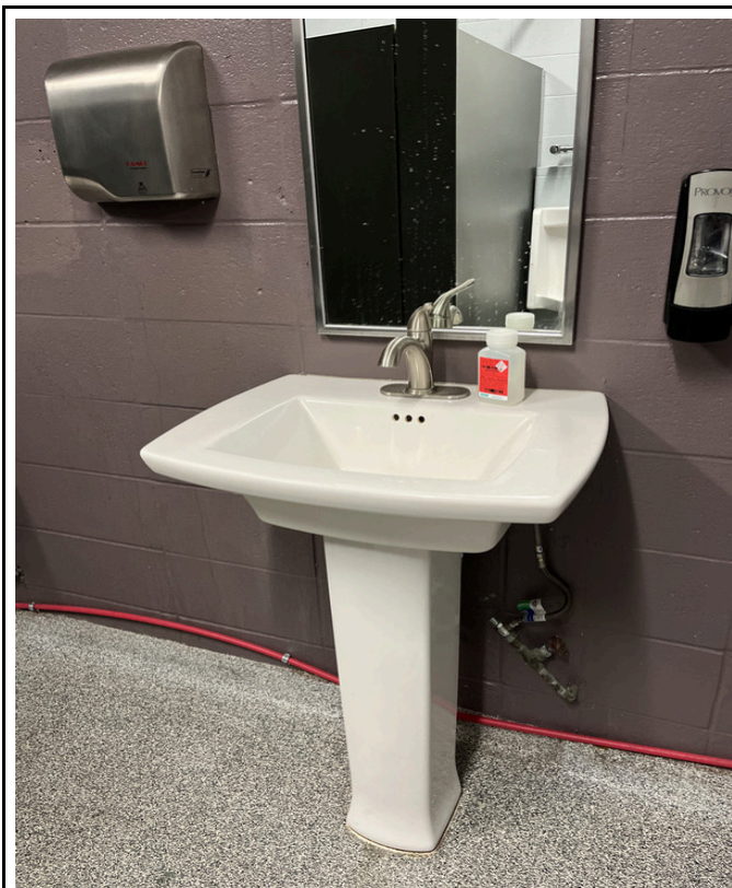
3/12/2024 - 5801-73 - Midway R-1 - Men's Restroom Across From Room 114 - Furthest From Door
