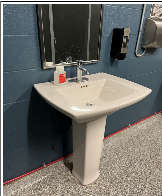
3/12/2024 - 5801-77 - Midway R-1 - Women's Restroom Across From Room 114 - Furthest From Door
