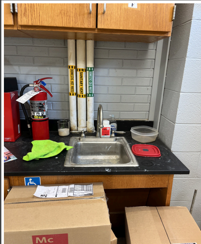
3/12/2024 - 5801-71 - Midway R-1 - Room 109 - East Wall
